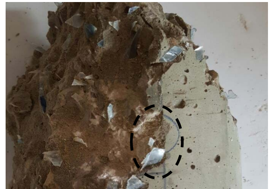
Figure 10 Concrete cylinder inspected after failure, showing the presence of PET flakes
